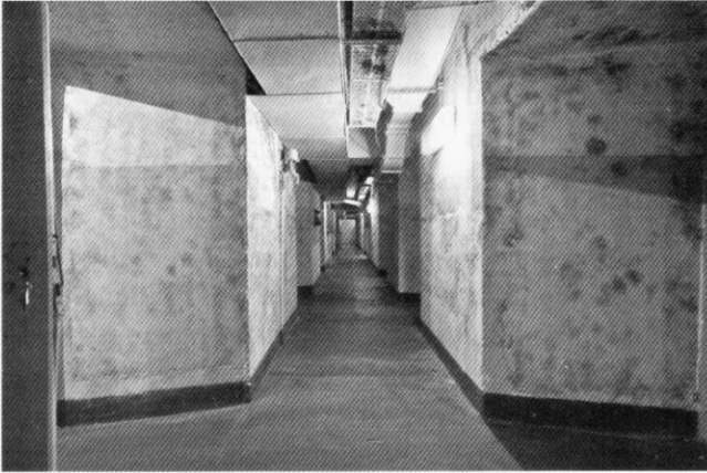
Upstairs, the corridor splits to the left and to the right leading to additional rooms. An alarm klaxon is on the wall in the middle of the picture
